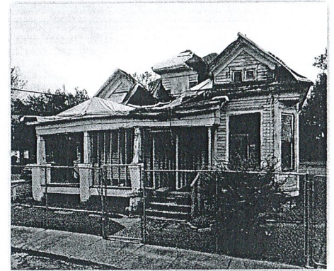
Lewis Home renovations 14
